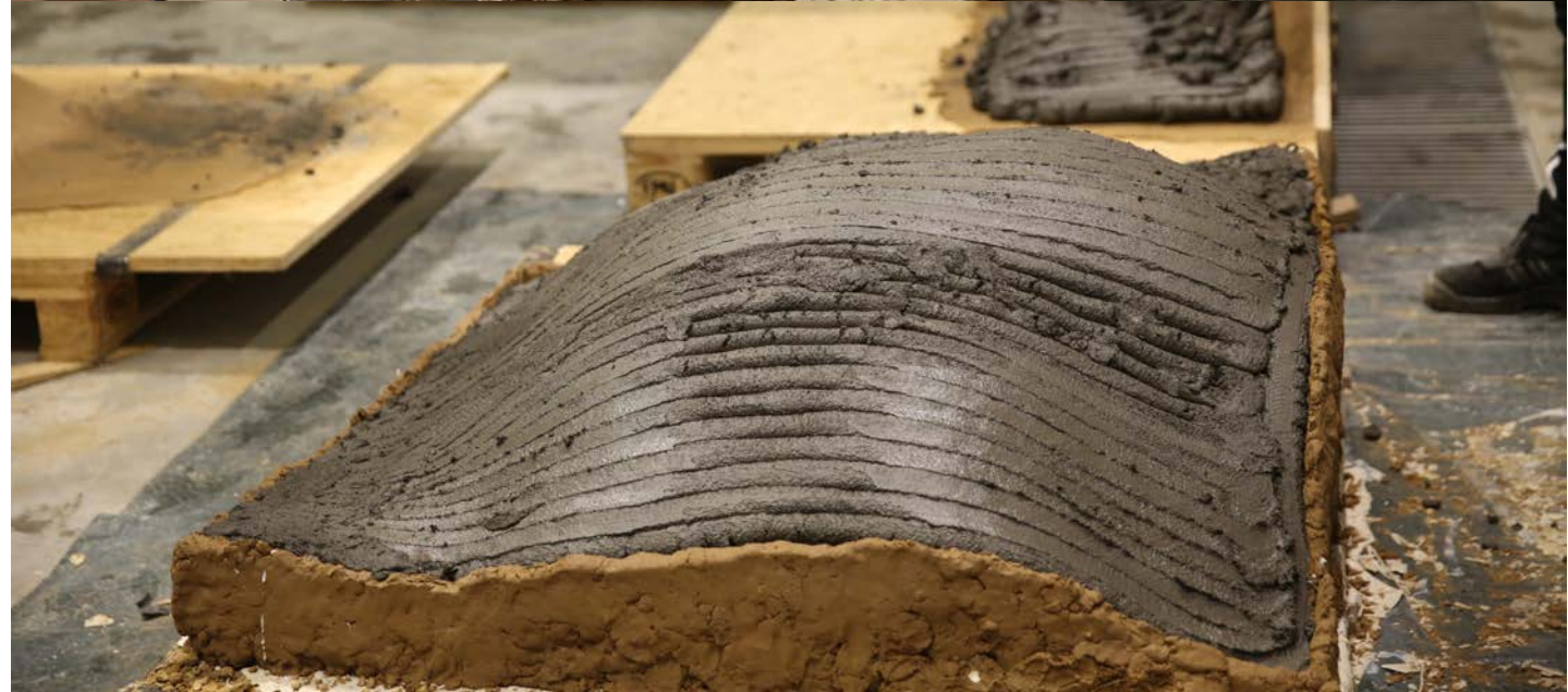
robotic concrete printing at TU-Braunschweig
